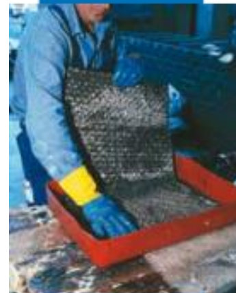
Manual impregnation of MapeWrap C
